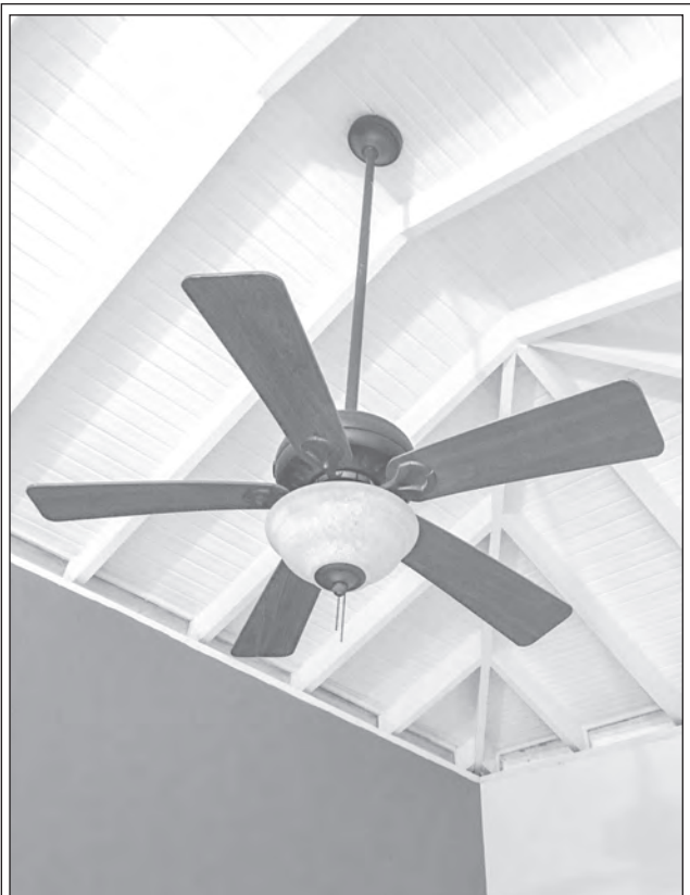
Contributed photo Reversing ceiling fans in winter can help redirect warm air from the ceiling into living spaces below.
