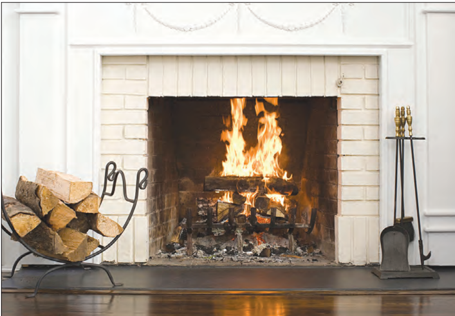
Contributed photo Neglect of chimneys and fireplaces can pose a range of notable dangers, including increased risk for carbon monoxide poisoning and chimney fires. Poorly maintained fireplaces also may fail prematurely, which is not insignificant, as a new fireplace can cost thousands of dollars.
