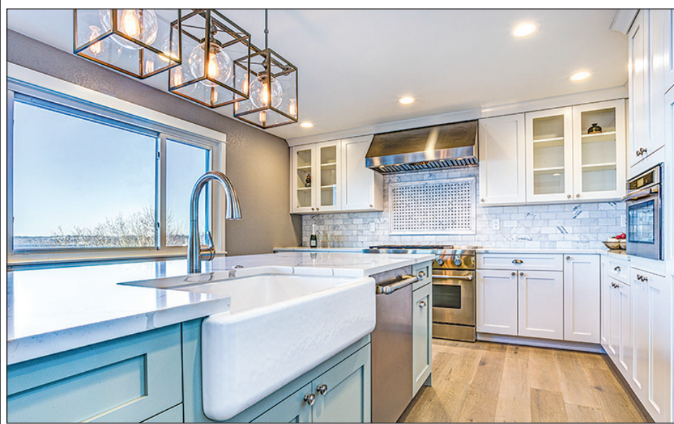
Cabinet replacement involves removing all of the existing cabinets before new cabinets are leveled and installed. According to the home improvement resource, The Spruce, homeowners can expect to pay between $13,000 and $30,000 for contractor-grade cabinets. Cabinet replacement is a good idea when homeowners want to add more cabinet space or create a new layout in the room.
